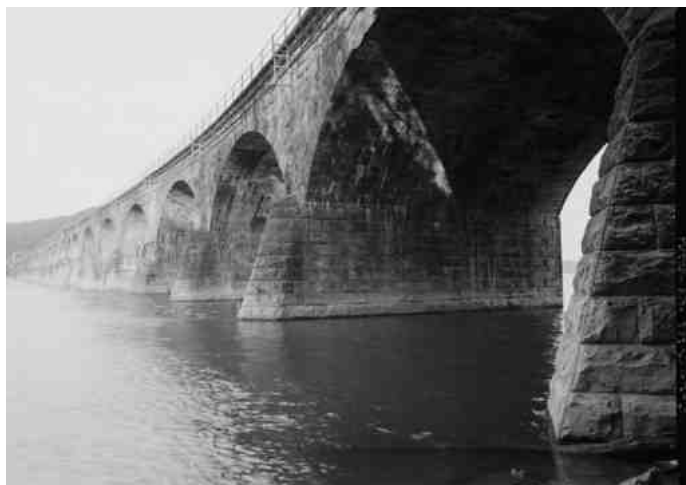
The Rockville Bridge spanning the Susquehanna River, north of I-81. Historic American Engineering Record, Prints & Photographs Division, Library of Congress, HAER PA, 22-ROCVI, 1.
